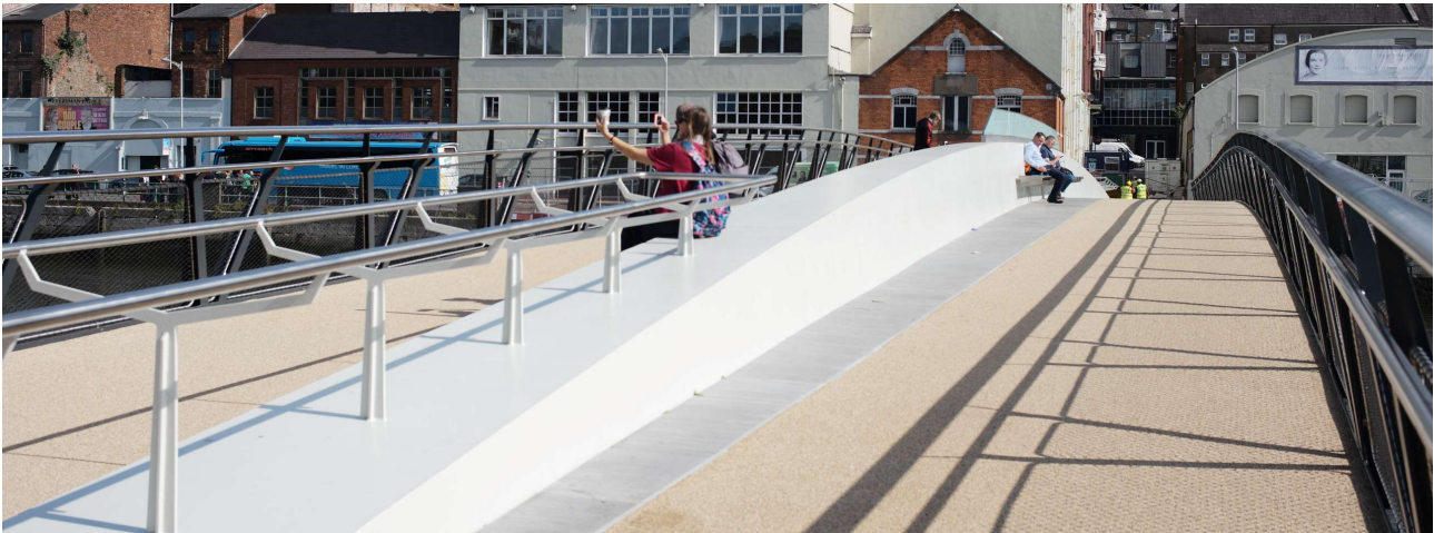
Fig. 17. Bridge View from the pedestrian path
