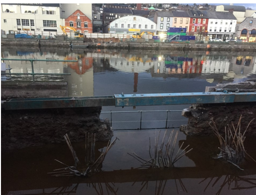
Fig. 15. Abutment construction and bridge being floated upstream to its final location
